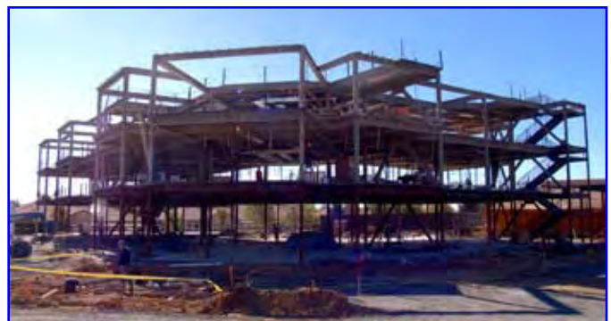
Assisted living building adds its fireproofing!
